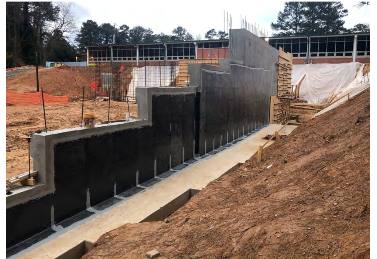
West Side of Gym Addition- Waterproofing
