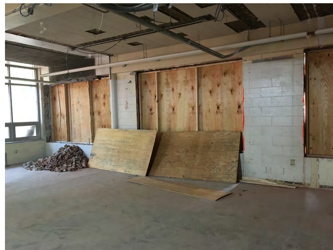
Openings for New Windows Cut in Existing Walls
